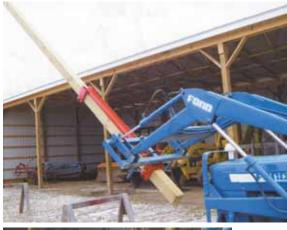
Photo shows 6 by 6-in. post being raised into position.
