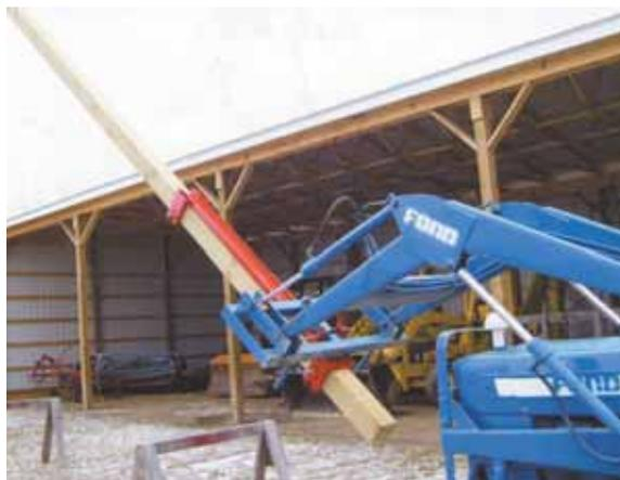
Photo shows 6 by 6-in. post being raised into position.
