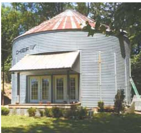
Previous owner of 40-ft. tall bin had cut a 14-ft. sq. hole in it for storage. The Weisers filled the hole with French doors and windows, then added a porch. They also added a second floor with stairway for more bedroom space. Kitchen is on first floor.
