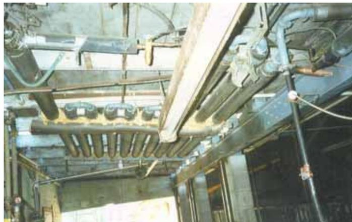
Pre-cooler was designed to mount against the ceiling, cooling milk down to 47 degrees.
