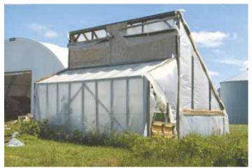
Hydroponic 12 by 20-ft. greenhouse is covered with heavy plastic. Sloping south roof maximizes sun warmth.
