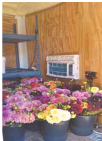
Raindrop Farms needed more storage for their fresh flower business, so they converted an 8 by 10-ft. cargo trailer into a mobile cooler that makes use of a window-style air conditioner controlled by a "Cool Bot".
