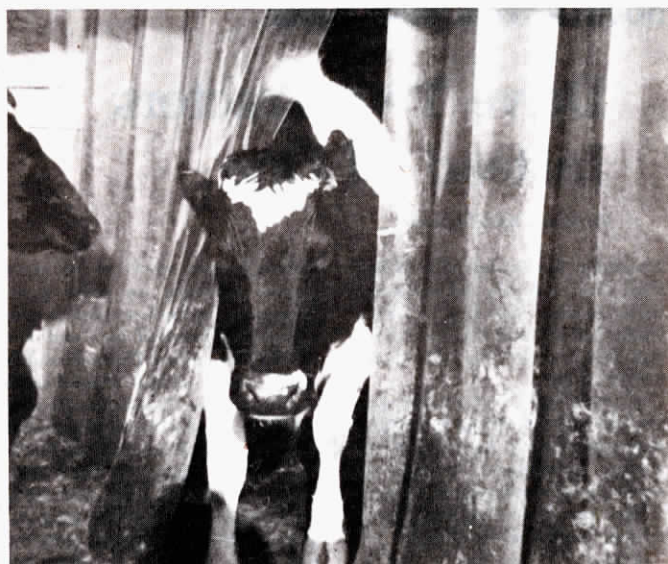
After animal passes through, strips fall back into place to seal opening. Typical installation uses 12 in. wide strips, with two-thirds overlap of the strips.
