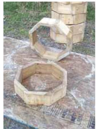
Octagon-shaped cement pad is lifted with a detachable metal handle. Colby uses 2 by 6 forms (right) to make the pads, which serve as footing for poles.
