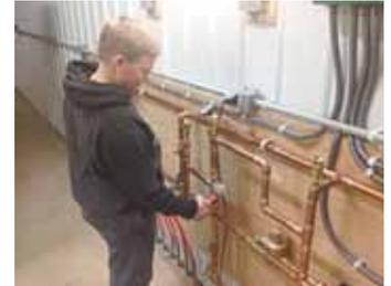
The Schetters designed and installed this manifold and hooked it up to a Log Boss wood-fired boiler.
