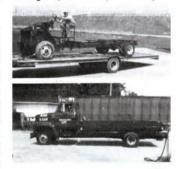
I bought a Ford motorhome chassis built in 1986 with no miles on it for \$4,000. It's powered by a 460 V-8 engine. I installed a 1976 International 2010 cab on the frame and aded a 14-ft. flatbed. I ended up with a good truck at a reasonable price. (Richard Hinds, 4271 Sangamon Ave. Rd., Springfleld, III. 62707)
