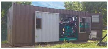
Mobile gasification plant consists of a 150 kW generator powered by a biomass gasifica-tion system, with everything tucked inside a 20-ft. long shipping container.
