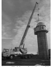
A crane lifted the gazebo to the top of the 36-ft. tall by 12-ft. dia. silo.
