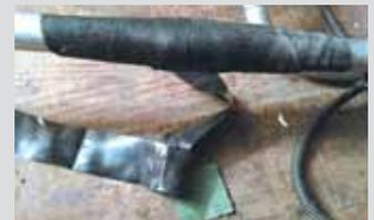
resin by rubbing it with the gloved hand. I then wrapped the tape tightly with the vinyl strip and left it for about 5 min.
