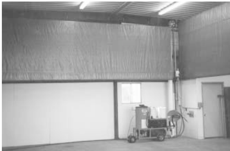
Curtain rolls up or down automatically and stores up out of the way near the rafters when it's not needed.
