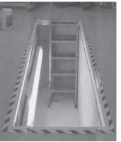
ft., 4 in. wide. I built a frame of 4 by 4-in. angle iron around the top edge to pour the slab against. It cost only \$350 more than a plain flat slab but it has already paid for itself in ease of maintenance on trucks, tractors, ATV's, and equipment.
