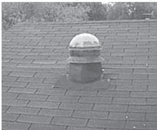
Co., ph 800 844-4786; www.sunpipe.com). "It's a solar tube that pulls light down from the roof. Of course it works only during daylight conditions but it eliminates the need to turn on the lights during the day. Nature pays the power bill. It consists of a silver-coated pipe 9, 13, or 21 inches in diameter with a dome on top and diffuser dome at the base. The pipe can be just about any length. It comes with good instructions for do-it-yourself installation and is reasonably priced."
