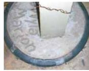
Vertical beam sets inside 6-ft. deep, 18-in. dia. hole lined by a ribbed poly culvert and filled with 2 ft. of concrete.
