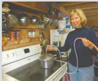
**Bernis Ingvaldson, The Honeyberry Farm, Bagley, Minn.:** "With little snow cover last winter, the water line from the well to our house froze. By connecting some tubing from the outlet on a pressure cooker into the water line, we were able to produce enough steam to thaw the pipe in no time, saving \$200 on a service call."
