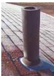
Frost-free sewer vent consists of 2 pieces of pipe with an air gap between them.
