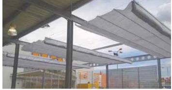
Roof uses a system of struts, cables and fabric screening strong enough for a person to stand on. Photo shows roof partially retracted.
