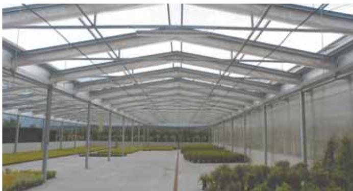
Novavert Retractable Roof can be closed quickly to protect plants against weather extremes. Photo shows roof completely retracted.
