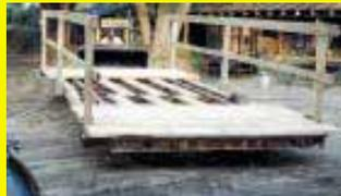
ft. long bridge that was designed for pedestrians, light vehicles and horse-drawn wagons, but he wanted it replaced. The steel-framed trailer had been used to carry a backhoe towed behind a dump truck. I removed the trailer's fenders and front and rear axles. I also cut the center axle from the frame and then chained it
