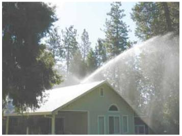
Roof Safer Sprinkler keeps roofs wet to prevent flying embers from igniting. Sprinkler covers an 80-ft. dia. circle
