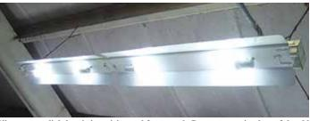
Kit uses your light's existing wiring and framework. Parts snap on in place of the old ballast cover.
