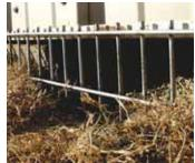
Underground animal barrier is made of 15-in. long, galvanized 4-ga. steel rods spaced 1 1/4 in. apart.
