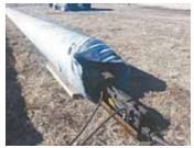
Scissors jack collapses to slip inside bent end of culvert.
