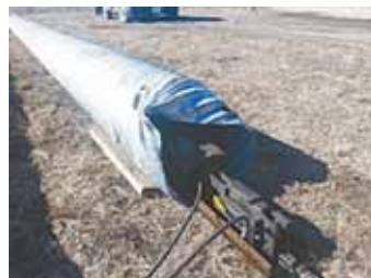
**Scissors jack collapses to slip inside bent end of culvert.**
