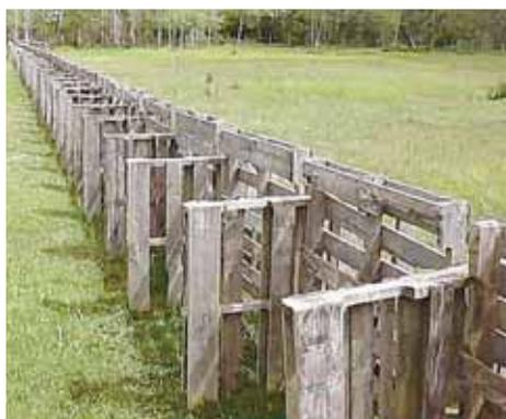
Pallets are used together at right angles.
