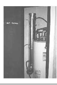
Cozy Heater mounts on side of any hot water heater and plumbs easily into the water lines.
