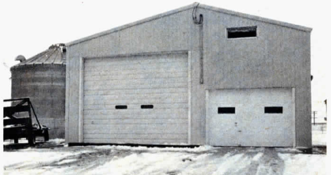
From outside, it looks like an ordinary machine shed. The large overhead door on left forms east wall of the living room.
