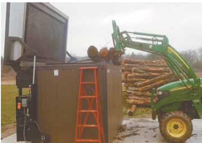
**Big firebox on Tom Lubbers's top loading wood boiler holds up to 1 3/4 cords of wood, in chunks up to 9 ft. long.**
