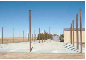
Doug Dumler used old center pivot pipe for the framing on his homebuilt, 60 by 60-ft. shed. Photo shows vertical pipes placed in cementfilled holes.
