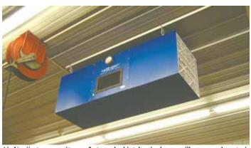
Air-Vac Systems says its new 5-stage, dual intake air cleaner will remove odors, toxic gases, chemical vapors, and also kill mold, bacteria and viruses.
