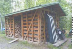
Heavybuilt shed has 4 by 4 corner posts with 2 by 6 wallboards spaced 8 in. apart.
