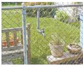
sell. I liked this one. The top rail of a chain link fence is a piece of galvanized pipe that's plumbed into a water line at the house and 3 water spigots spaced every 20 ft. around the yard for watering plants and grass. That way you don't have to drag a hose all over the yard."
