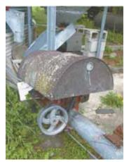
**David Obrecht, Zearing, Jowa:** To protect the electric motor on his bin auger from the weather, David cut a 55-gal. drum in half and mounted it over the top of the motor.
