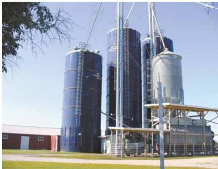
Michigan farmer Mark Hinterman converted two 20 by 70-ft. Harvestore silos to hold 18,000 bu. of grain each. He also converted a 20 by 50-ft. silo to hold 12,500 bu. for cooling grain after it goes through the dryer. Note holding bin next to silos.
