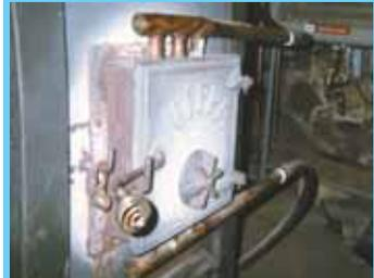
Tim Ojala built this removable hot water booster for his indoor wood stove. Three rows of U-shaped, 3/4-in. brass pipes heat the water.
