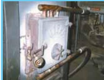
Tim Ojala built this removable hot water booster for his indoor wood stove. Three rows of U-shaped, 3/4-in. brass pipes heat the water.
