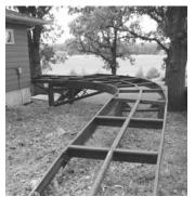
Stringers for the deck flooring are made with channel iron, I-beams and tubular steel that's welded in place.
