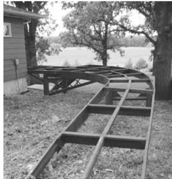
Stringers for the deck flooring are made with channel iron, I-beams and tubular steel that's welded in place.
