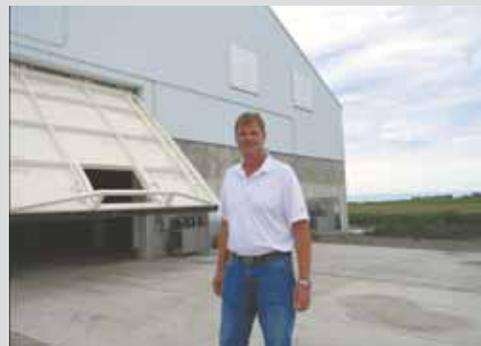
Hydraulic door installed on Tom Revier's 120 by 200-ft. feed storage building contains a 54 by 44-in. sliding door, which allows grain to pour out for augering into feed trucks.
