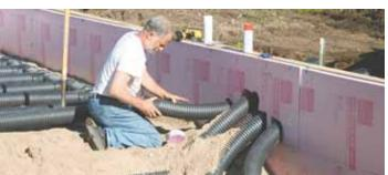
An in-line fan is used to push/pull air through the closed system of 4-in. corrugated
