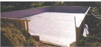
Staus prepared the base for the greenhouse by excavating 4 ft. of soil and laying down 2-in. rigid Styrofoam panels.
