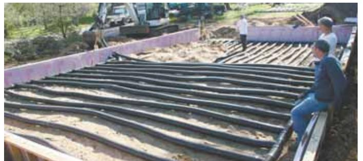
He laid one layer of heat tubes over the insulation. They were covered with sand, then a second layer of tubes was laid perpendicular to the first.
