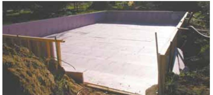
Staus prepared the base for the greenhouse by excavating 4 ft. of soil and laying down 2-in. rigid Styrofoam panels.
