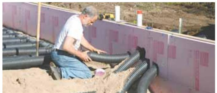
An in-line fan is used to push/pull air through the closed system of 4-in. corrugated drain tiles.
