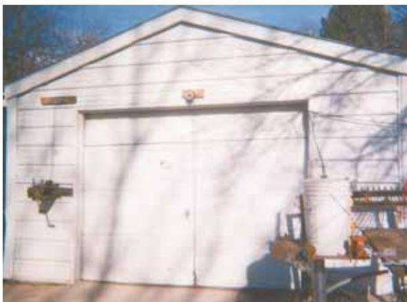
Hand-operated winch on one side of garage door is used to open door.
