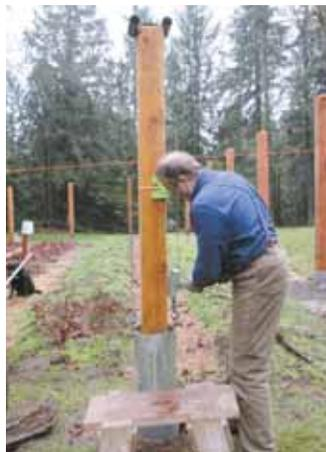
Come-along is used to pull metal duct out of hole, leaving landscape fabric in place.
