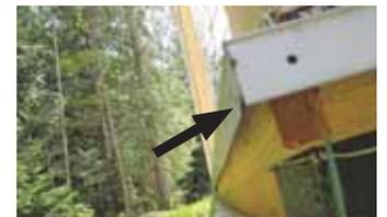
Slugs can't negotiate the turn at the bottom of this "slug fence" built from 2 by 6-in. metal "corner bead".
