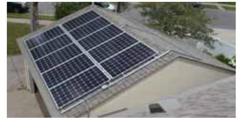
“No roof penetration” solar system (Solar Pod™ Crown).
