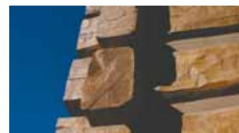
Concrete logs have the look and feel of real wood, right down to the grain, knots and growth rings that appear on interior and exterior surfaces.
