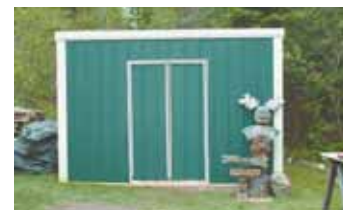
Steve Hoolsema built this 8 by 12-ft. building out of pallets after realizing that a purchased 12 by 12-ft. shed could cost him as much as $2,000.
