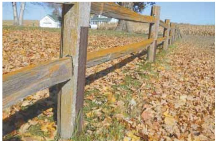
Loran Bauer uses steel posts to repair his split rail fence. He drives the post into the ground next to a weakened upright and then screws it in place.
